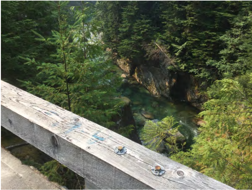
Looking downstream from deck
