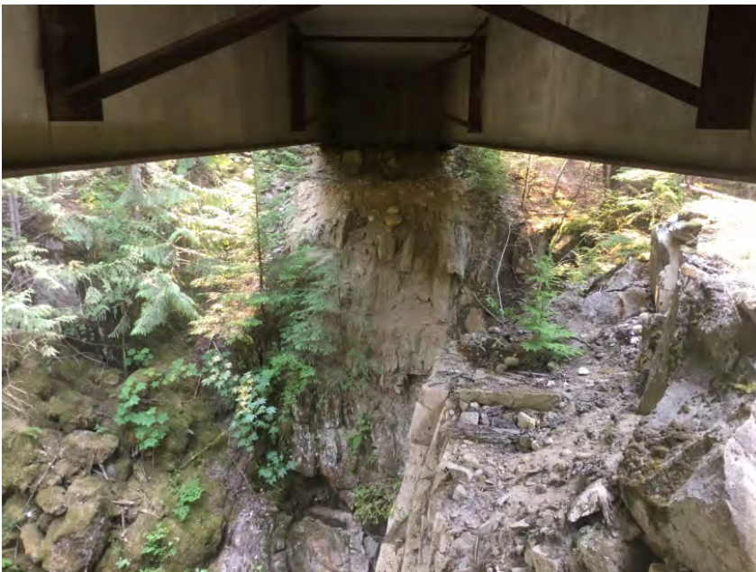
Left Bank Abutment when facing downstream
