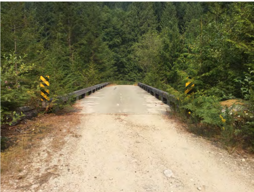
Approach from Left Bank when facing downstream
