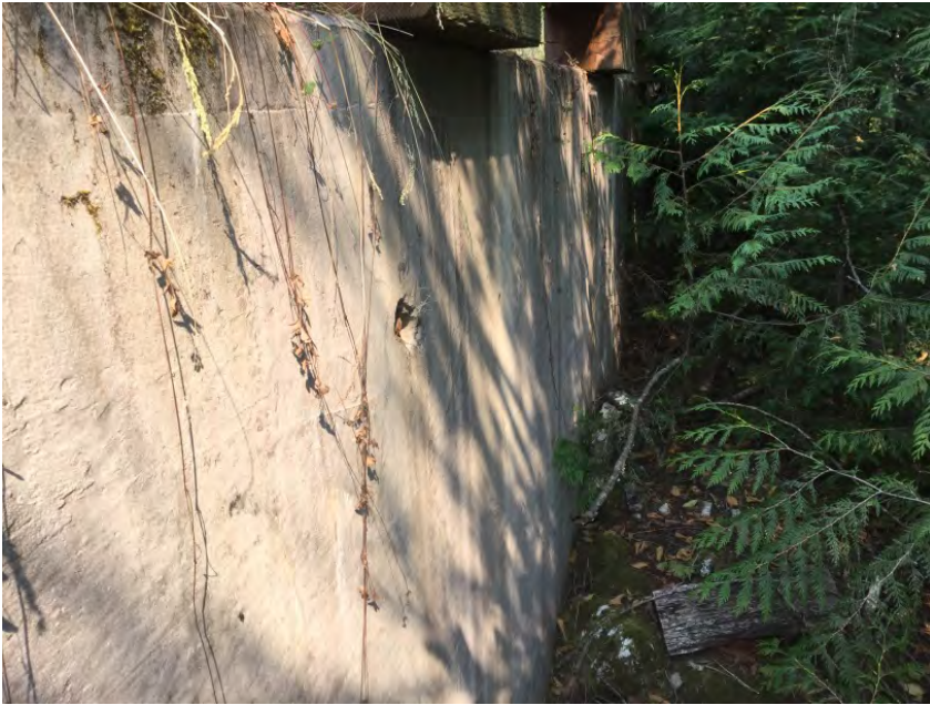
Upstream right bank wingwall - 1 piece precast concrete
