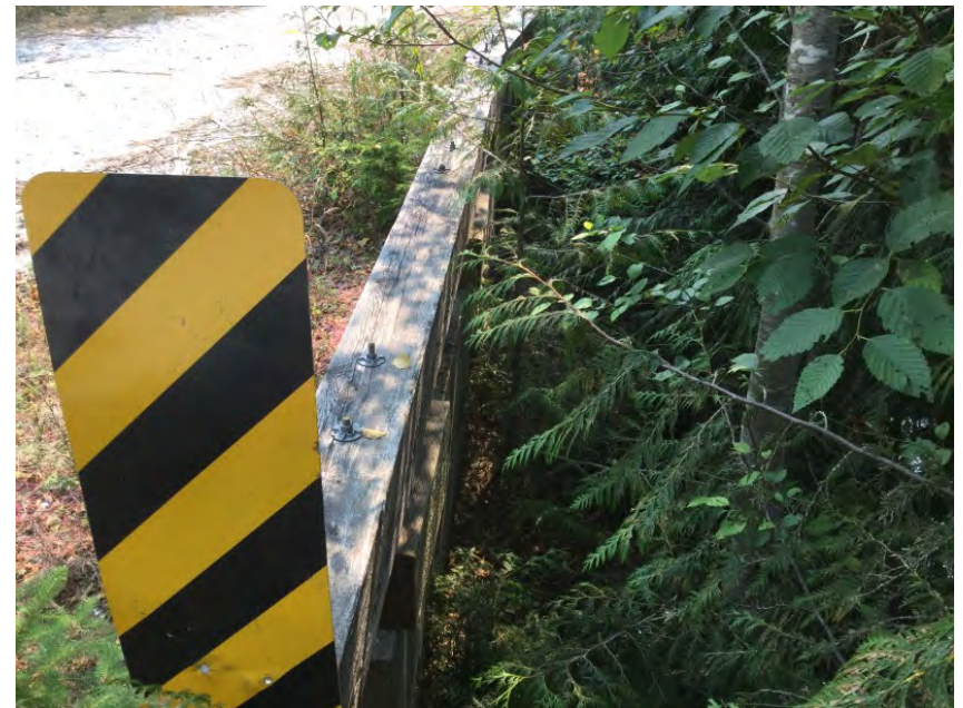
Downstream right bank wingwall - 3 piece precast concrete
