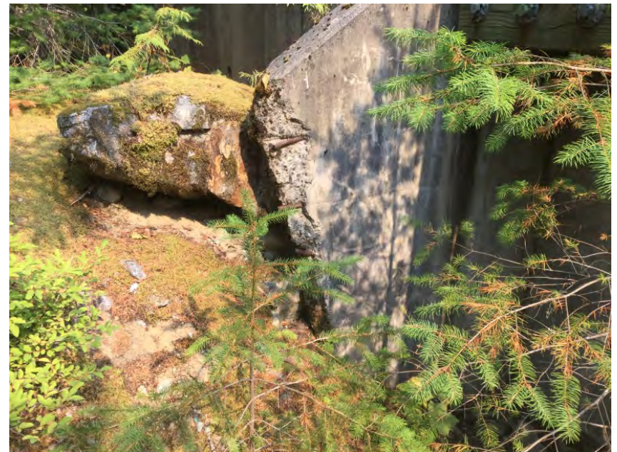
Downstream right bank portion of ballast wall removed due to terrain feature
