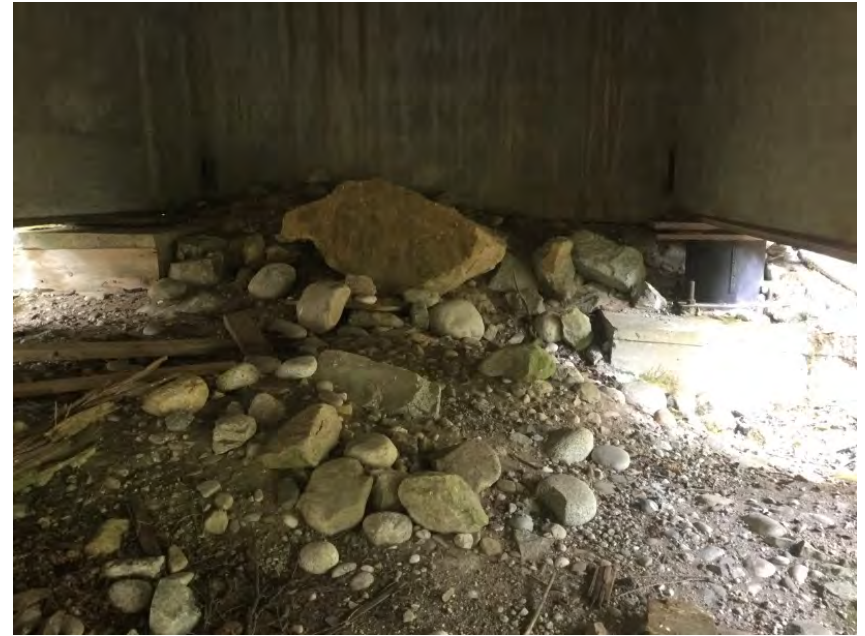
Right Bank Abutment when facing downstream
