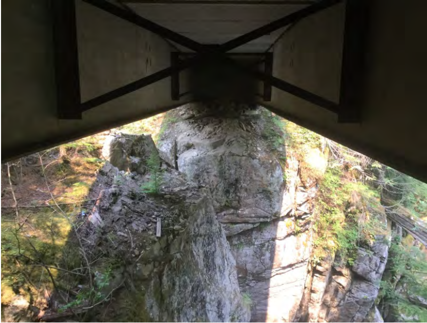
Right Bank Abutment when facing downstream
